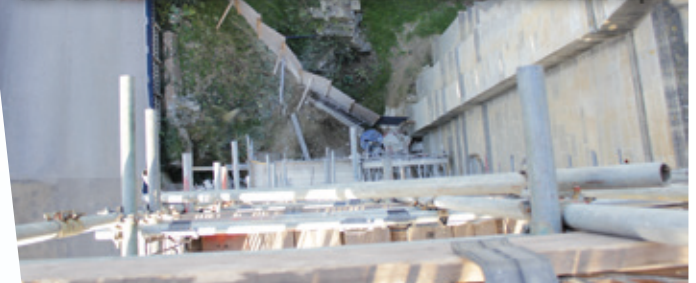
The north-west foundation viewed from the scaffold top.
