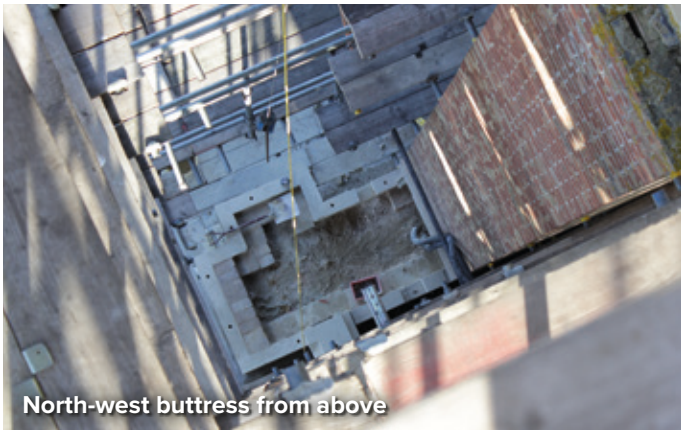
Stone, brick core and limecrete centre in the north-west buttress
